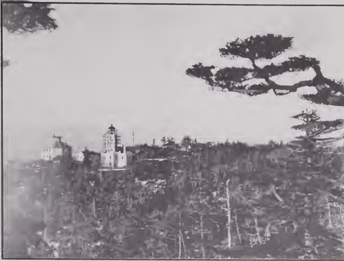
Opposite page: Erosion approaches the original Cape Hinchinbrook, 1933. Left: Construction of the new lighthouse is nearly complete in 1934.
