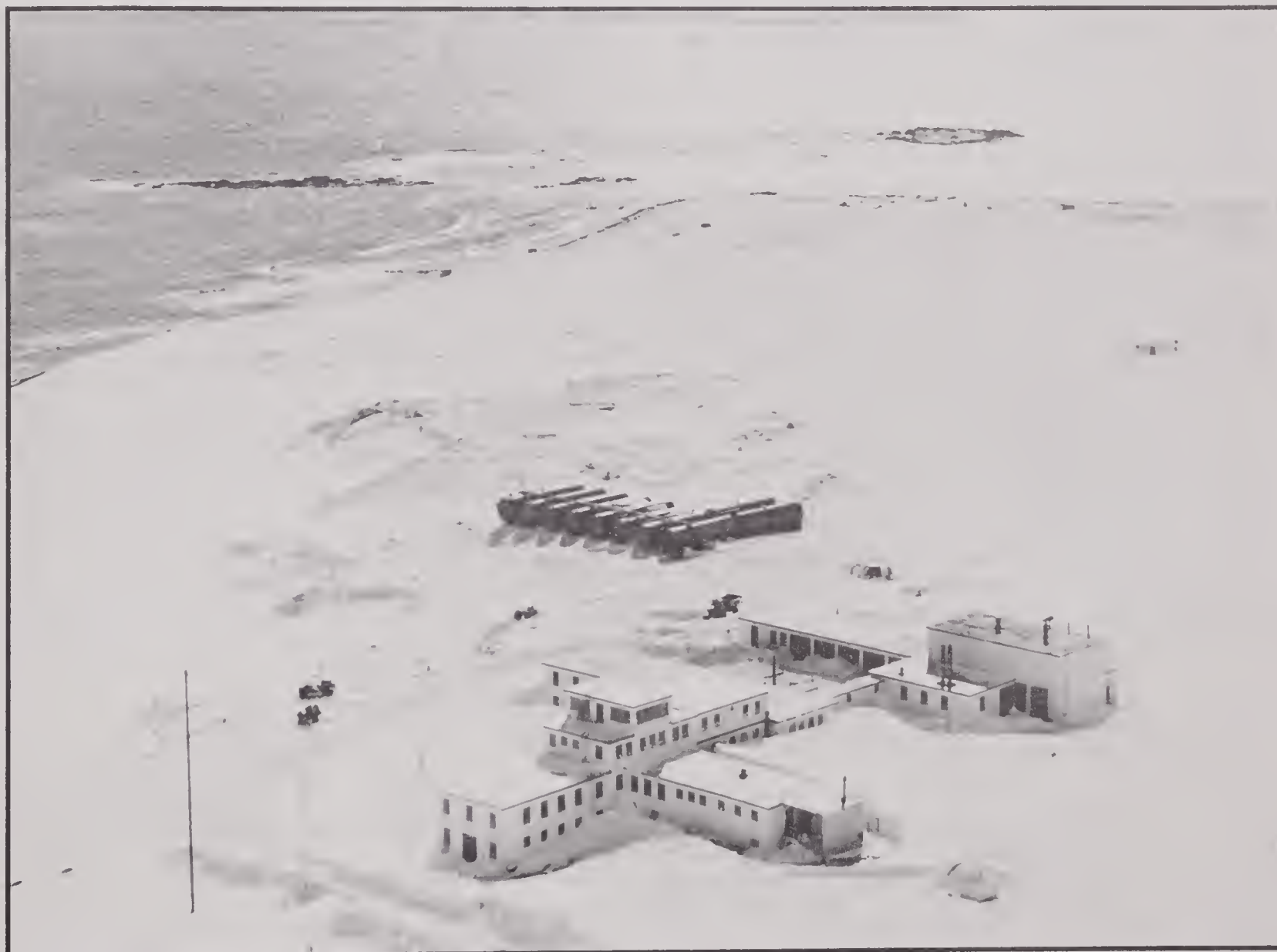
Loran Station Attu, located on the last island of the Aleutians, was commissioned in the 1960s.
