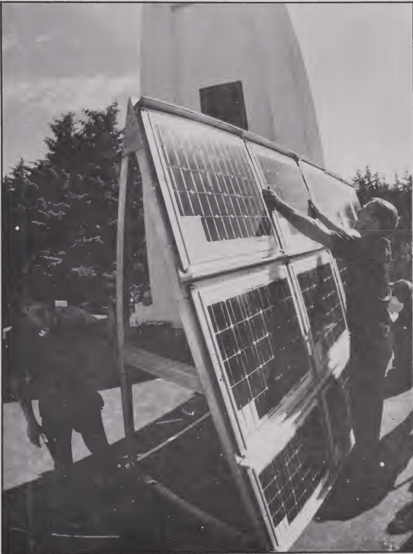
Left: Sentinel Island's wharf and boat-house, June 21, 1915. Below: The lighthouse is modernized with the installation of solar panels to reduce the need for generators, and to cut maintenance costs.
