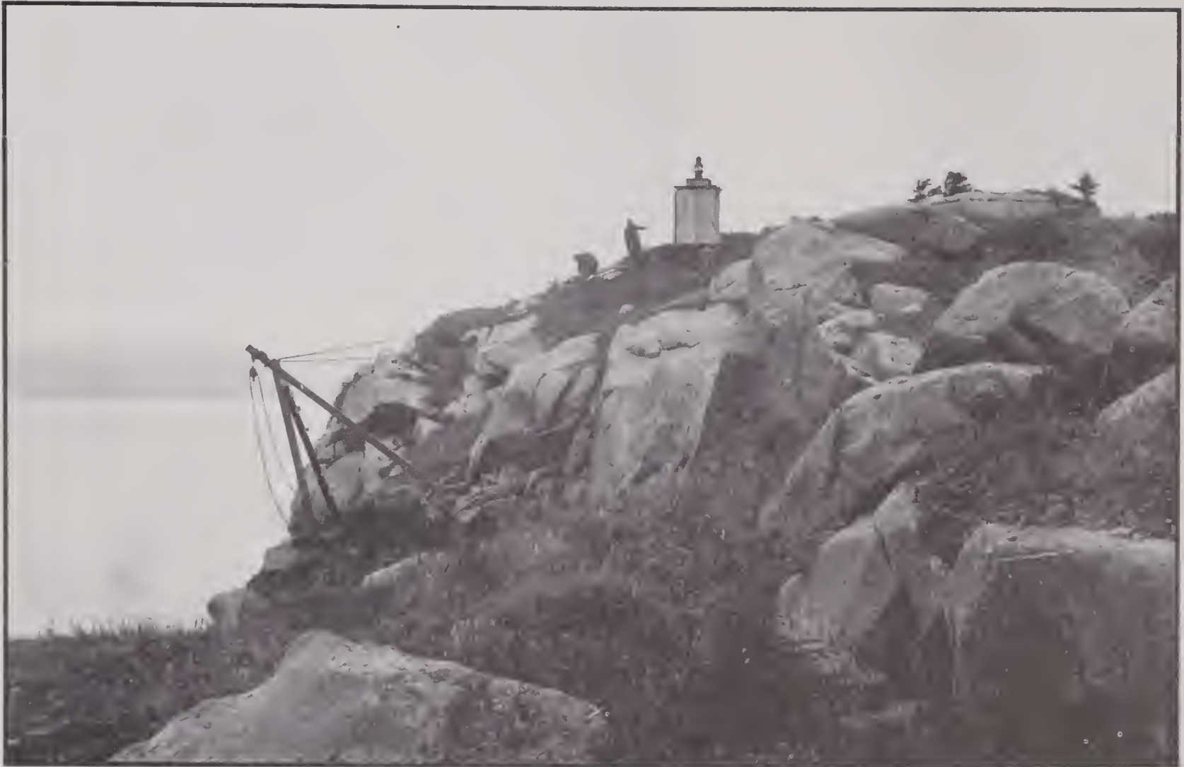
Rugged Island Light at the entrance to Resurrection Bay. An aid is still on the site.
