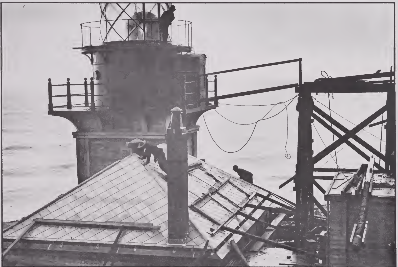
Construction of Cape St. Elias Light Station began in 1915.
