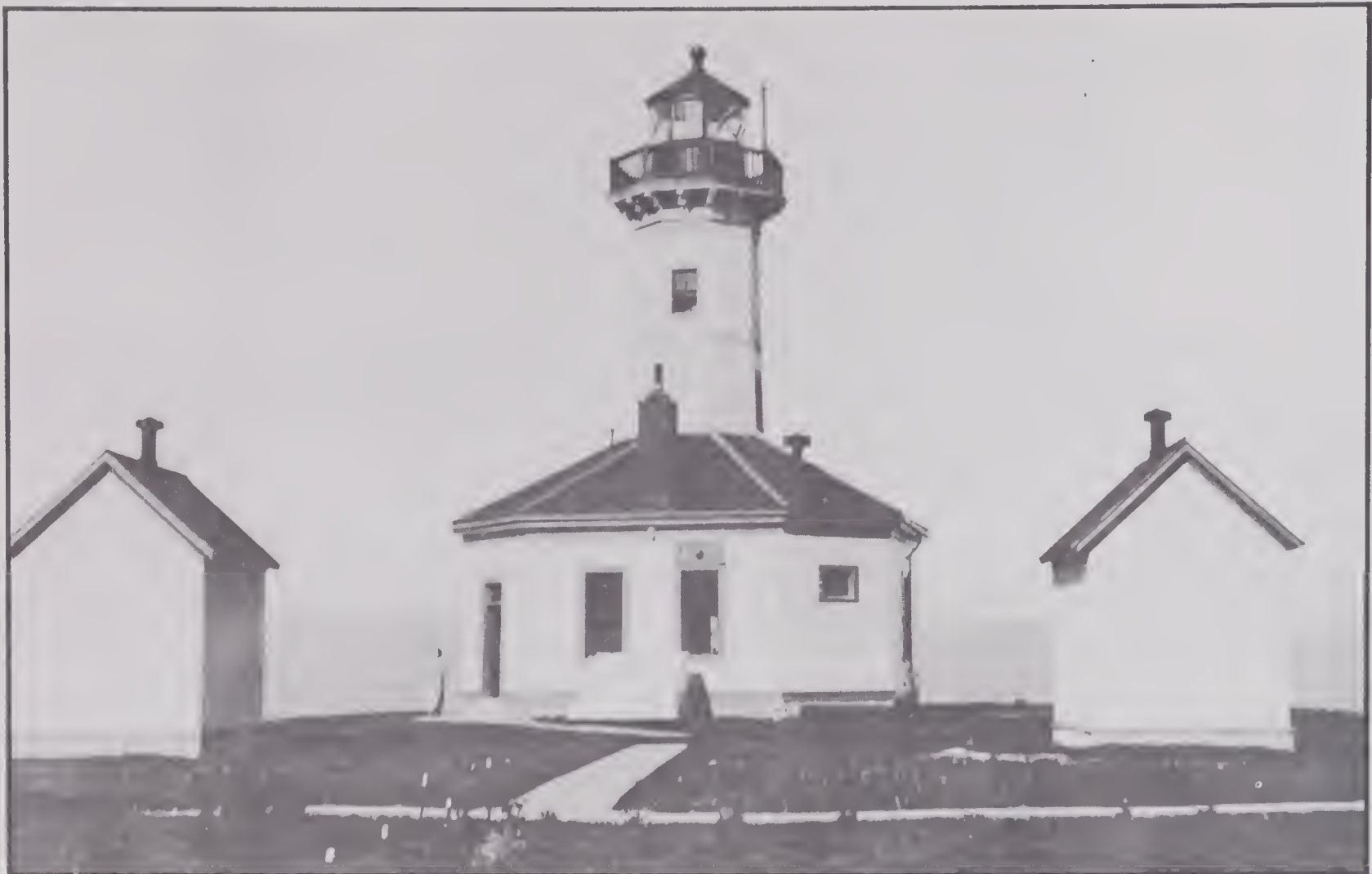
The original lighthouse structure at Mary Island.
